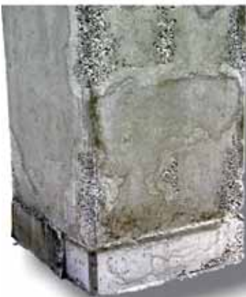
With high-cycle vibration in congested rebar
