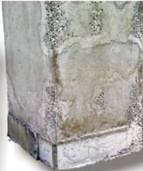
With high-cycle vibration in congested rebar
