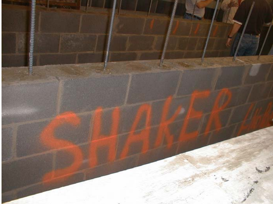
Figure 1. Completed wall prior to testing
